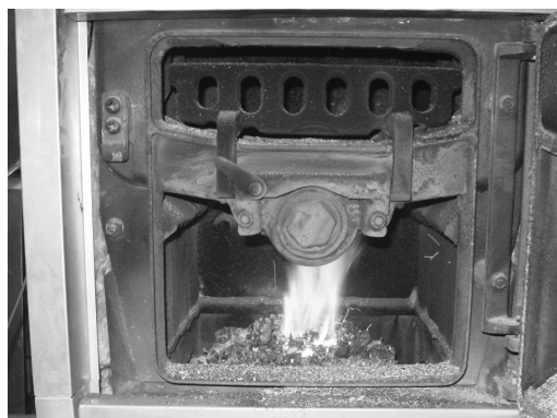
Fig.No. 28 Awkward shape of the flame
